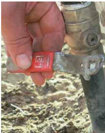
*It pays to install a globe valve on the water supply to the trough so the valve can be easily serviced, or the trough can be turned off. Note the valve handle has been removed to prevent cattle accidentally shutting off the trough. The valve can be operated using fencing pliers, or by using the old handle as a spanner.*
